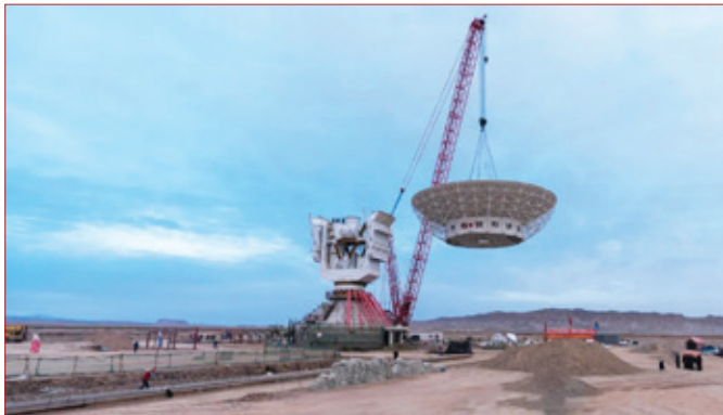
The 1 st of the 35-m Kashi antennas under construction. Credit: Lu Long / Kashgar Observation and Control Station
